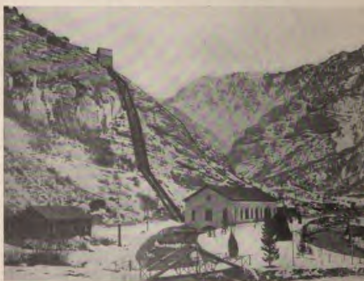
FIG. 6.—THE LOGAN POWER-HOUSE.
